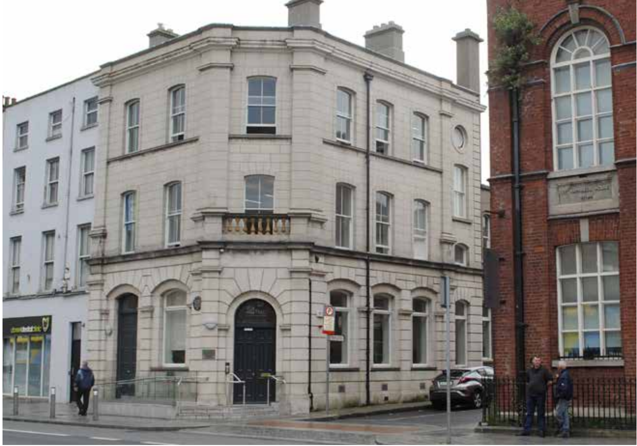
FLAC's Offices at 85/86 Dorset Street Upper.
